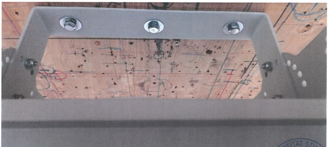
Figure 2 Detail: suspension of the installation element "SPACE-2-S"
